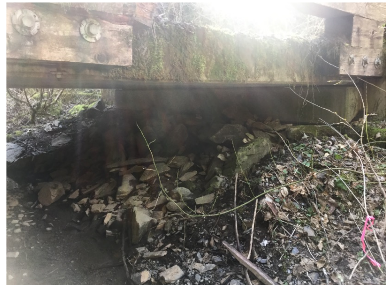
Left Bank Abutment when facing downstream
