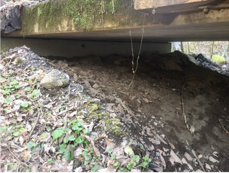
Right Bank Abutment when facing downstream
